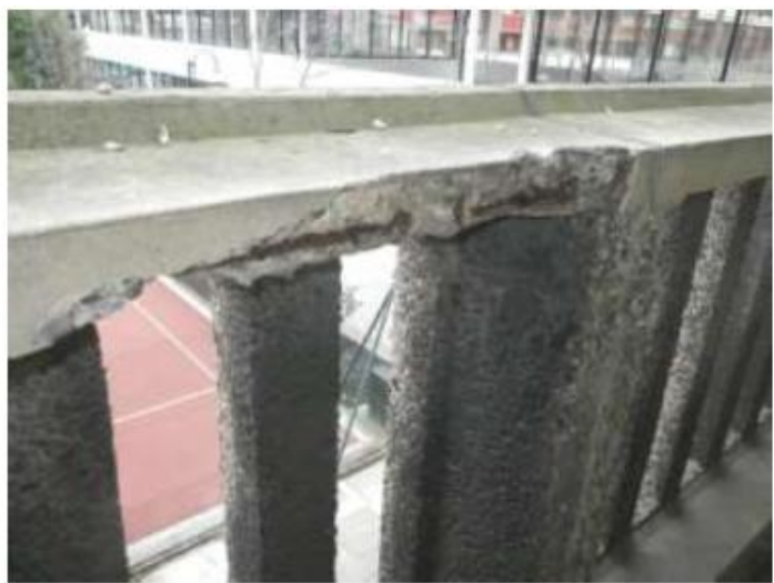
Photographs 2a and 2b: North Elevation, Cullum Welch House. Showing damage to vertical bars of balustrade and to a cill after removal of loose concrete. Photographs were taken before the installation of safety netting.
