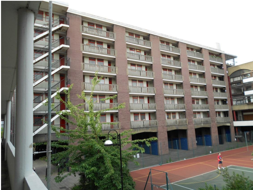
Photograph 1: North Elevation, Cullum Welch House. Showing balustrades and external staircase.
