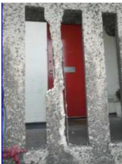
Photographs 2a and 2b: North Elevation, Cullum Welch House. Showing damage to vertical bars of balustrade and to a cill after removal of loose concrete. Photographs were taken before the installation of safety netting.
